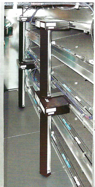
Dynamic 2" Super V-Banks and Sterile Sweep UVC Systems provide state-of-the-art air filtration, while reducing HVAC fan energy costs and extending maintenance intervals.
